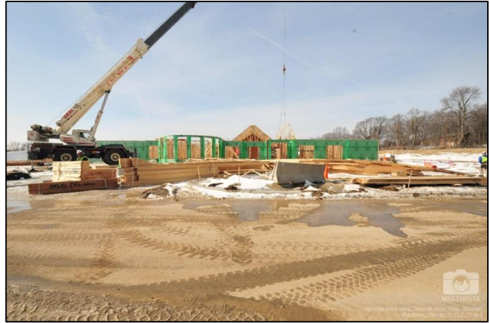
Figure 5 – Roof Truss Construction
