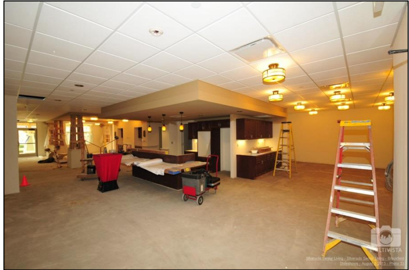
Figure 6 – Interior Light Fixture Installation
