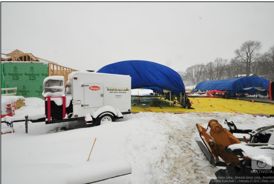
Figure 9 – Cold Weather Concrete Placement
